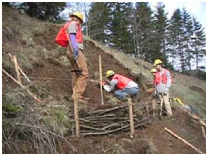
Figure 740.13 Leveling Line for the Next Willow Fence
