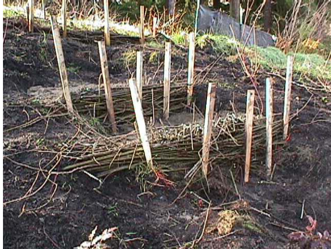
Figure 740.15 Live Gully Repair
