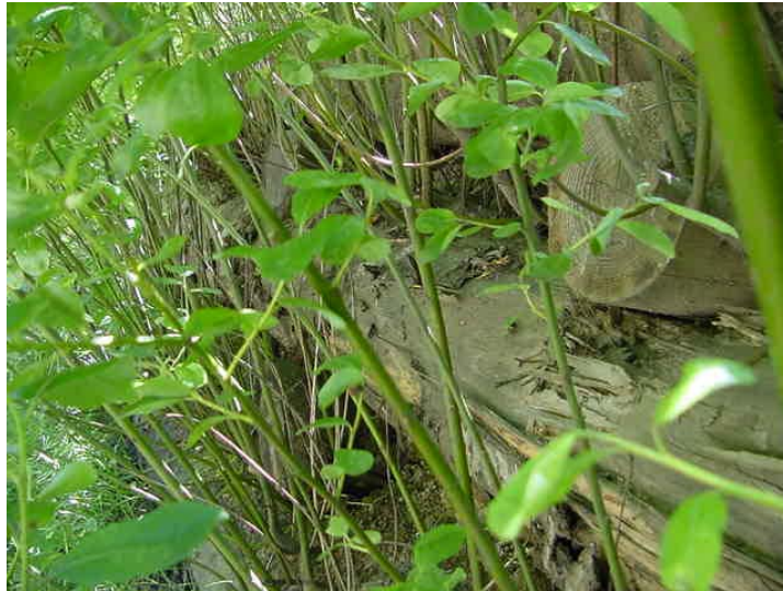
Figure 740.7 Live Cribwall 18 months after installation
