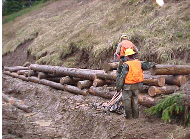
Figure 740.5 Live Cribwall Under Construction
