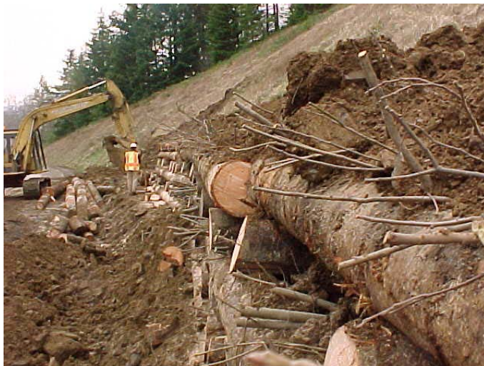
Figure 740.6 Live Cribwall with Willow Stakes
