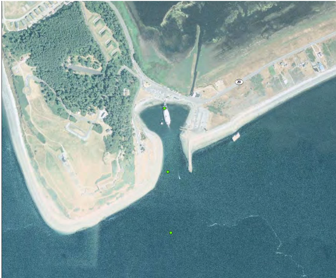
Figure 1: Location of near field and far field monitoring locations at the Keystone Ferry Terminal.
