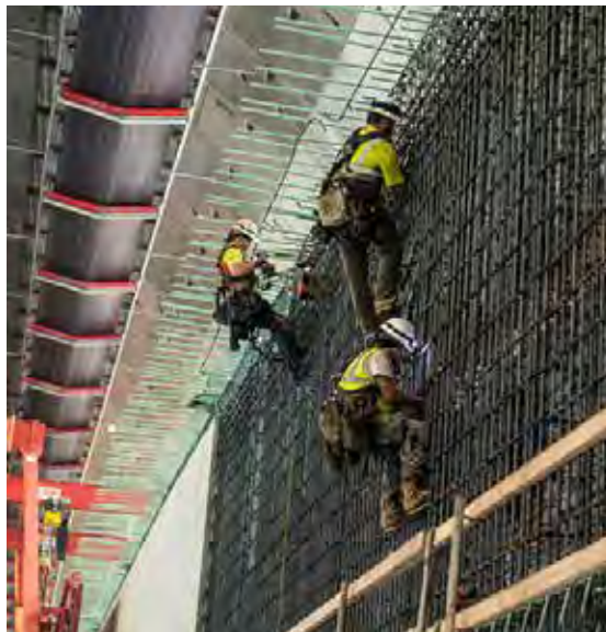
Building the roadway inside the tunnel
