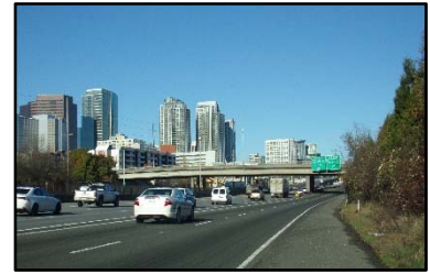
Existing Main Street Overpass
