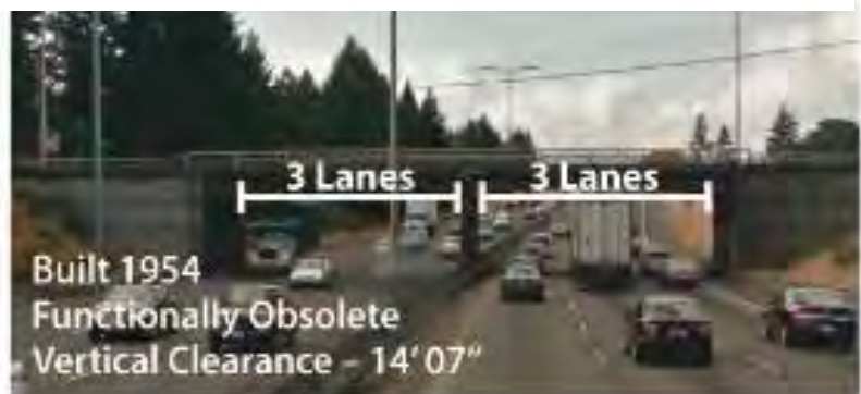
Figure PP1-12: Thorne Lane Bridge
