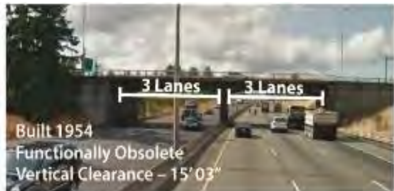
Figure PP1-11: Berkeley Street Bridge
