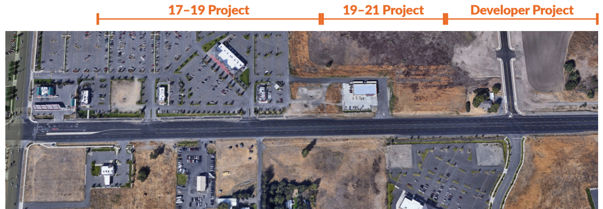
This project channelized the median between the eastern end of the 17-19 project and the Deer Heights developer project. WSDOT provided $110,000 in funding to the developer for this project, as part of the Deer Heights roundabout, after they completed the roundabout. The contractor used the project area for the traffic shifts.
