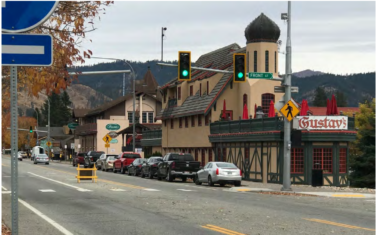
The new pedestrian crossing signal system on US 2 in Leavenworth
