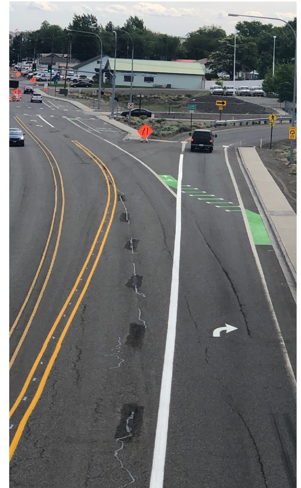
After: SR 240 with new left-turn pocket and drop lanes.
