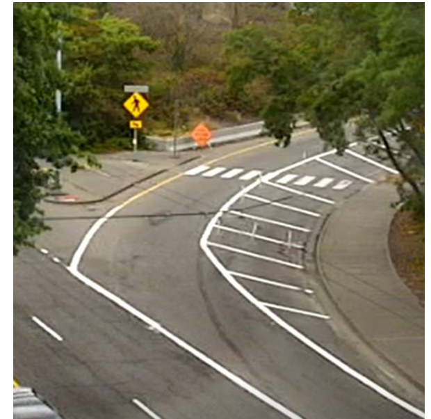
After: ramp reduced to a single-lane entrance with a metered shoulder downstream of the striping
