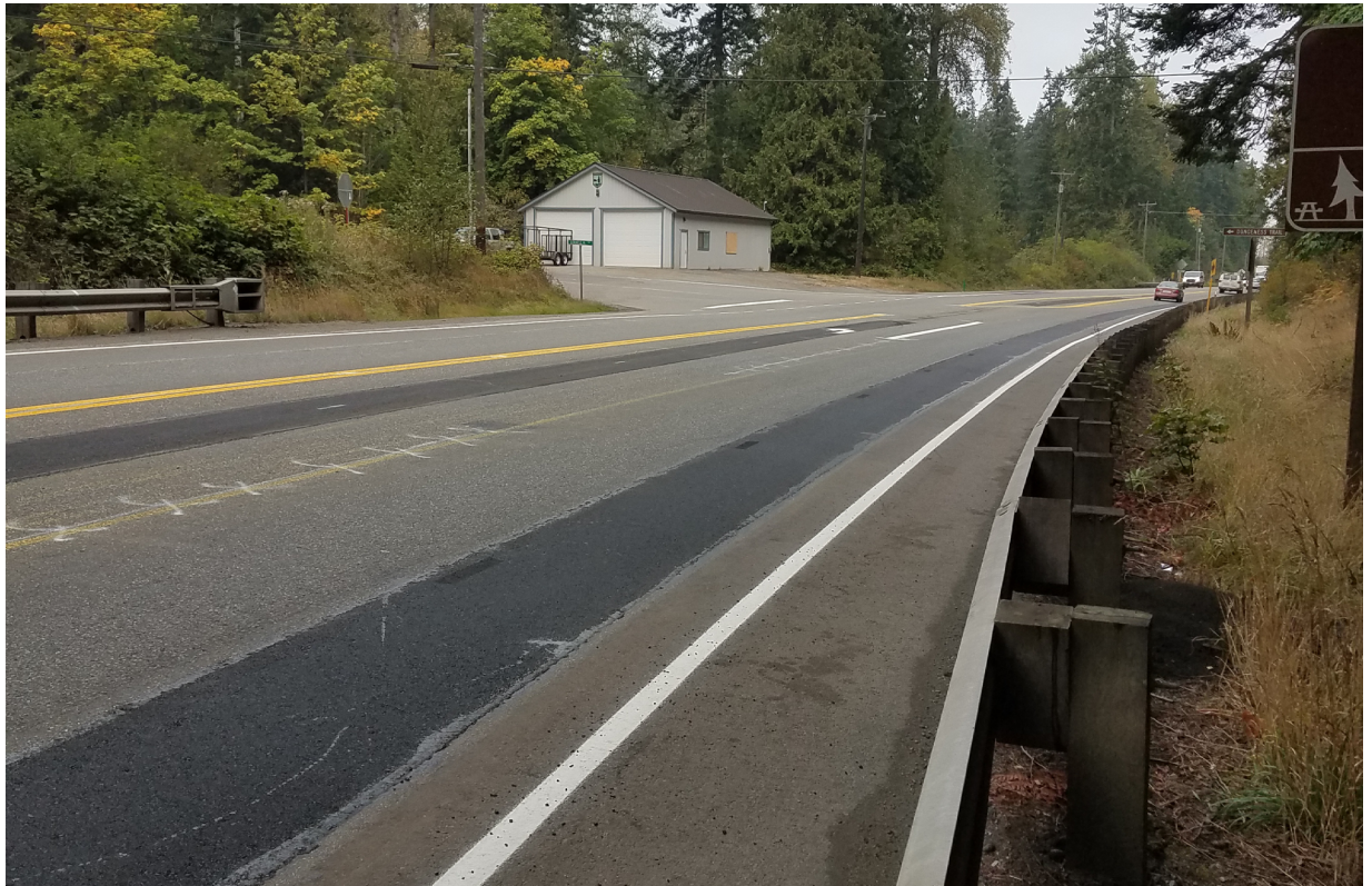
New left-turn lane on northbound US 101 at Louella Rd.
