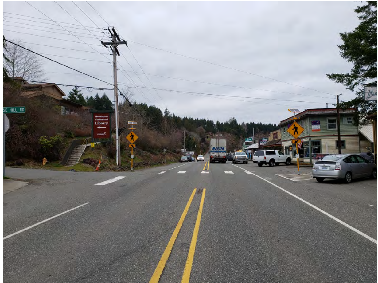
New Rectangular Rapid Flashing Beacons on US 101 in Hoodsport.
