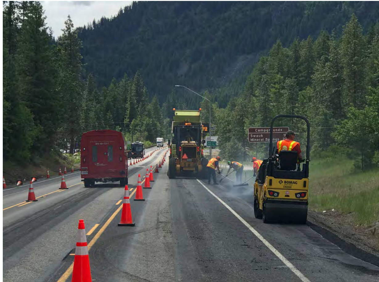
US 97 during installation of two-way left turn lane and restriping
